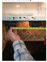
Repeat steps 3 & 4 to align and install the Right Auto-Out Microwave (marked R) on the right side of the microwave. Measure to ensure you have a minimum of 9.5" from center of Left unit to center of Right unit.
