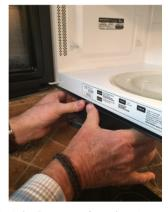
Slide Quick-Connect bracket into place between the bottom of the microwave and the metal panel (where space was just created by loosening the screws); push in until the bracket is flush with the edge of the panel. 5
